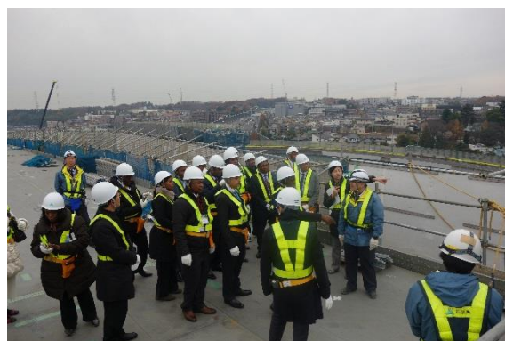
<Visit to Junction under Construction>
