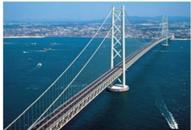
Akashi Bridge (Suspension Bridge)
