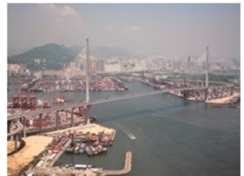
Stonecutters Bridge (Cable-Stayed Bridge, Hong Kong)
