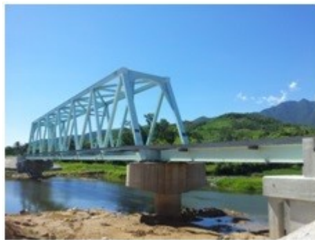
Railway Bridge (Truss, Vietnam)
