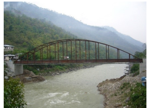
Sunkosh Bridge (Langer Bridge, Bhutan)
