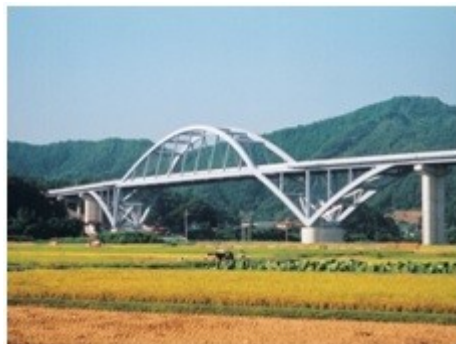
Maizuru-Yuragawa Bridge (Arch, Japan)
