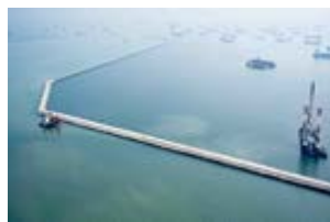
Port Rehabilitation (Indonesia)
