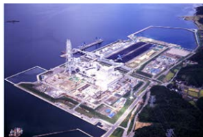
Power Plant (Japan)
