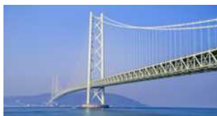
Social Infrastructure & Offshore Facilities
