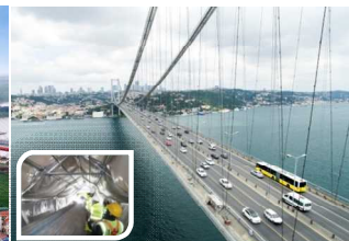
Rehabilitation Work 1st & 2nd Bosphorus Bridge Rehabilitation Project / Turkey
