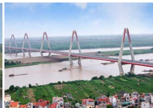
Cable-stayed Bridge NhatTan Bridge Vietnam
