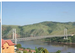
Suspension Bridge Matadi Bridge Project Democratic Republic of the Congo
