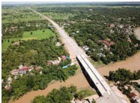
Improvement of National Road No.5 (North Section CP1) 【CAMBODIA】
