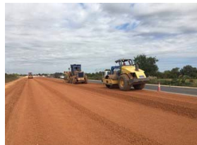
Improvement of National Road No.5 (Middle Section CP3) 【CAMBODIA】
