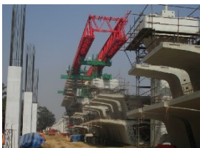
Dhaka Mass Rapid Transit Line-6 (CP5) Viaduct 【BANGLADESH】
