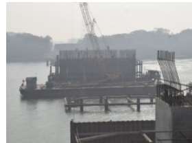
Cross Border Road Network Improvement Project Contract Package A1 【BANGLADESH】
