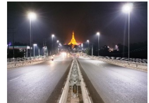
Infrastructure Development Project in Thilawa Area Phase II (Access Road Project) 【MYANMAR】
