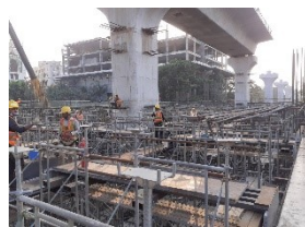
Dhaka Mass Rapid Transit Line-6 (CP5) Station 【BANGLADESH】
